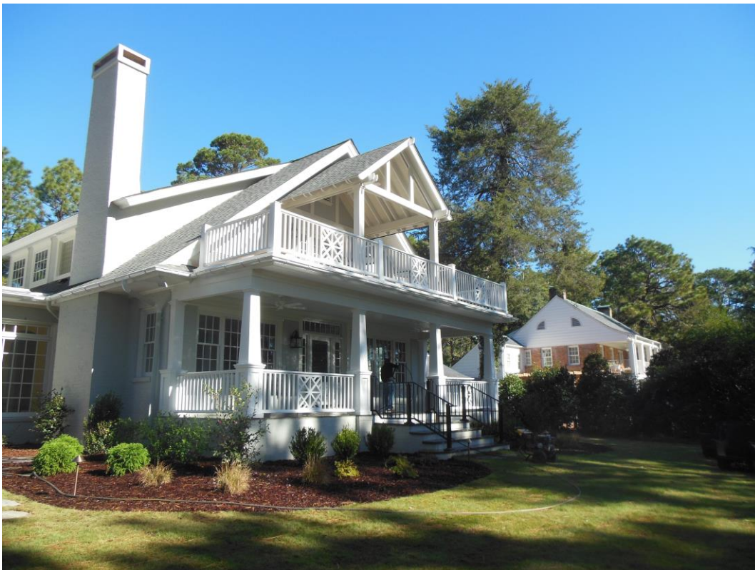
Rear porch and balcony addition
