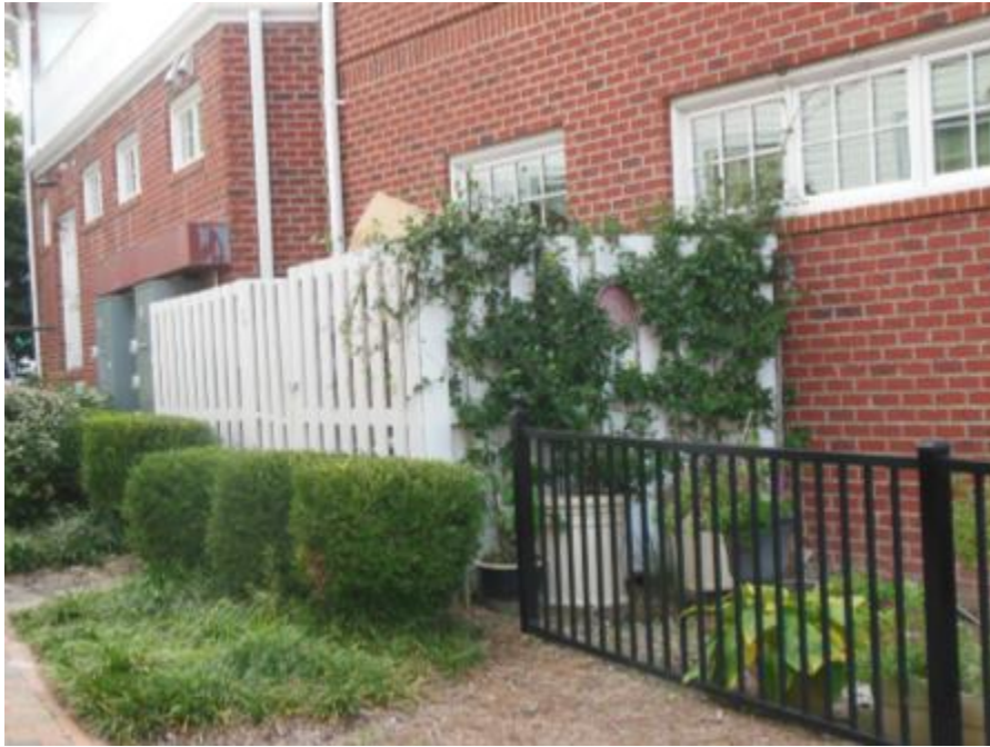
Screened commercial utility area
