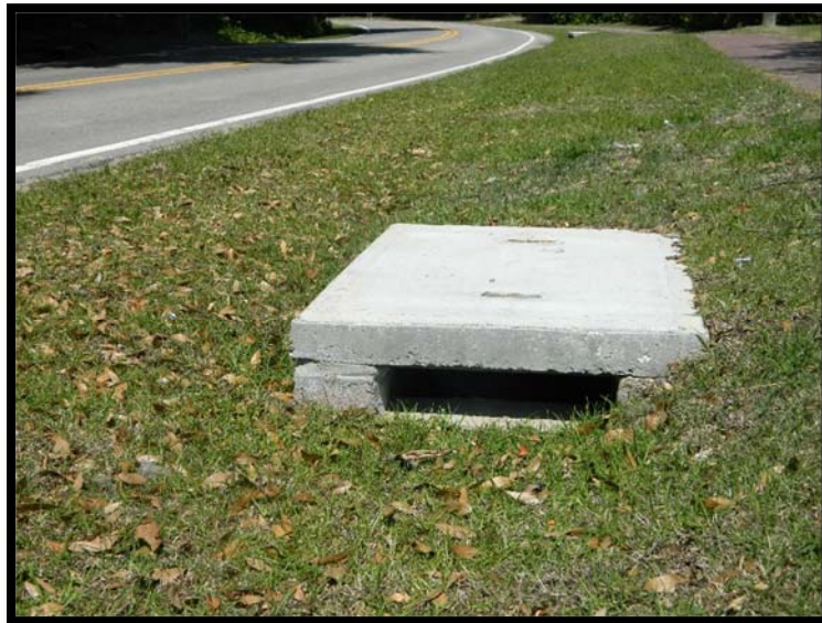
Stormwater improvement project
