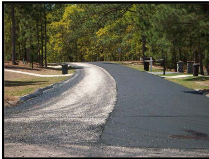
Village Street Resurfacing
