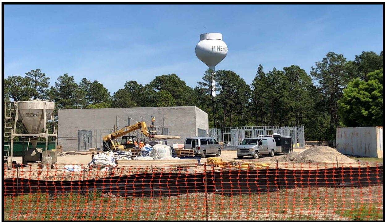
Community Center at Cannon Park Construction
