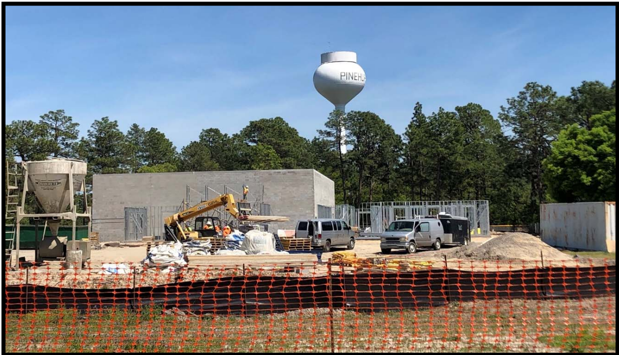
Community Center at Cannon Park Construction
