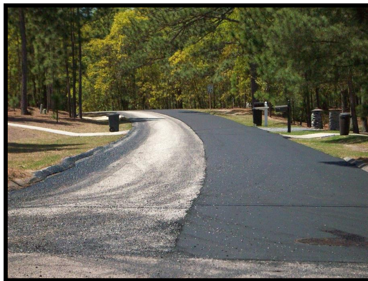
Village Street Resurfacing
