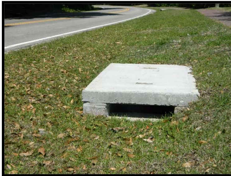
Stormwater improvement project
