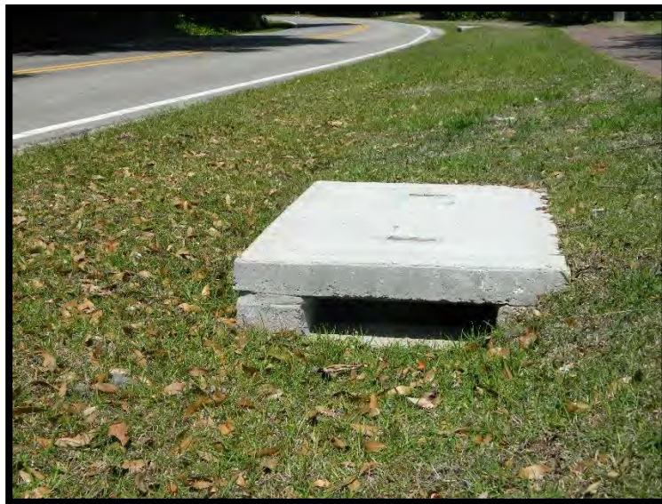
Stormwater improvement project
