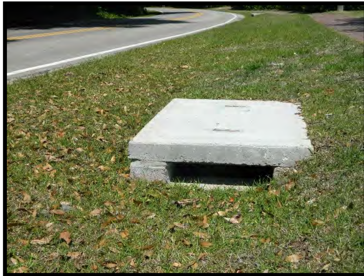
Stormwater improvement project
