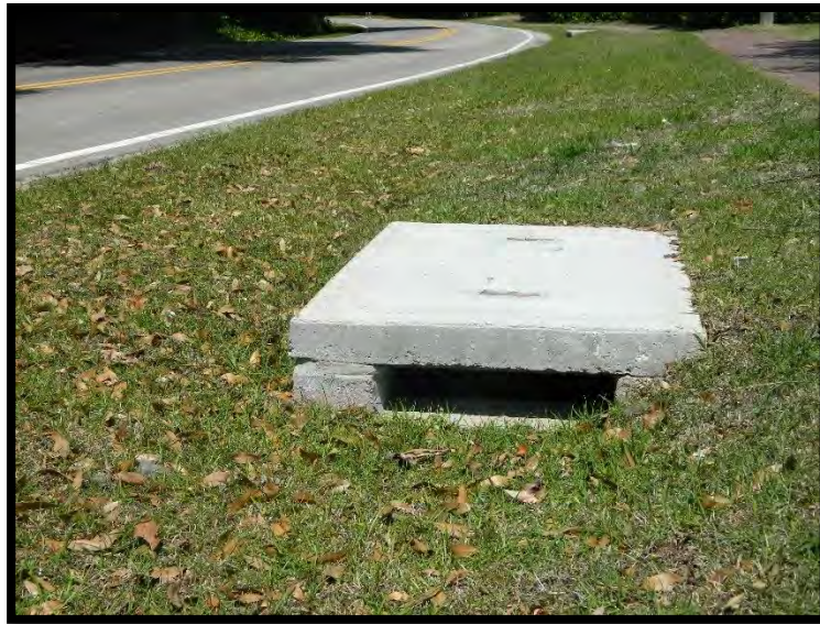
Stormwater improvement project
