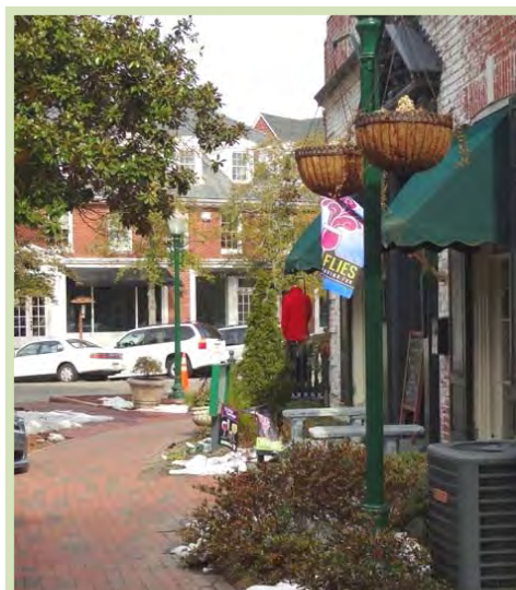
Install new and extend existing brick sidewalks in Village
