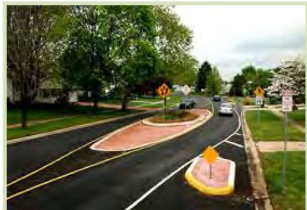
Chicanes are a set of 2 or 3 bulb-outs or curves that alternate from one side of the street to the other. They are designed to slow the speed of drivers – in this case, by creating a narrower lane.
