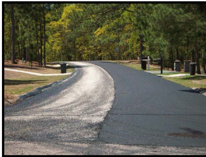
Village Street Resurfacing
