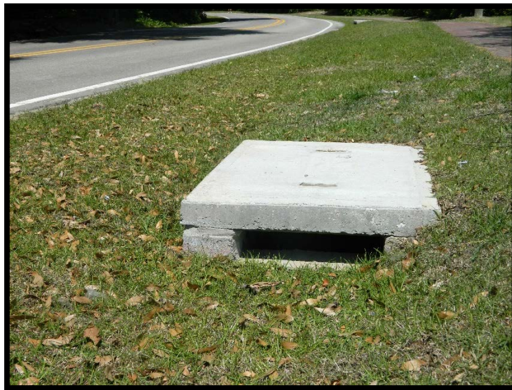
Stormwater improvement project
