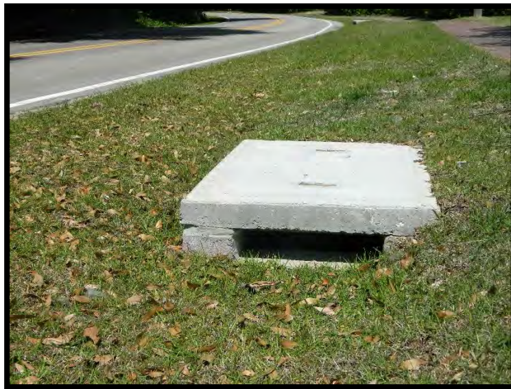
Stormwater improvement project
