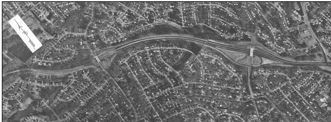
Benjamin Parkway after construction in 1990
