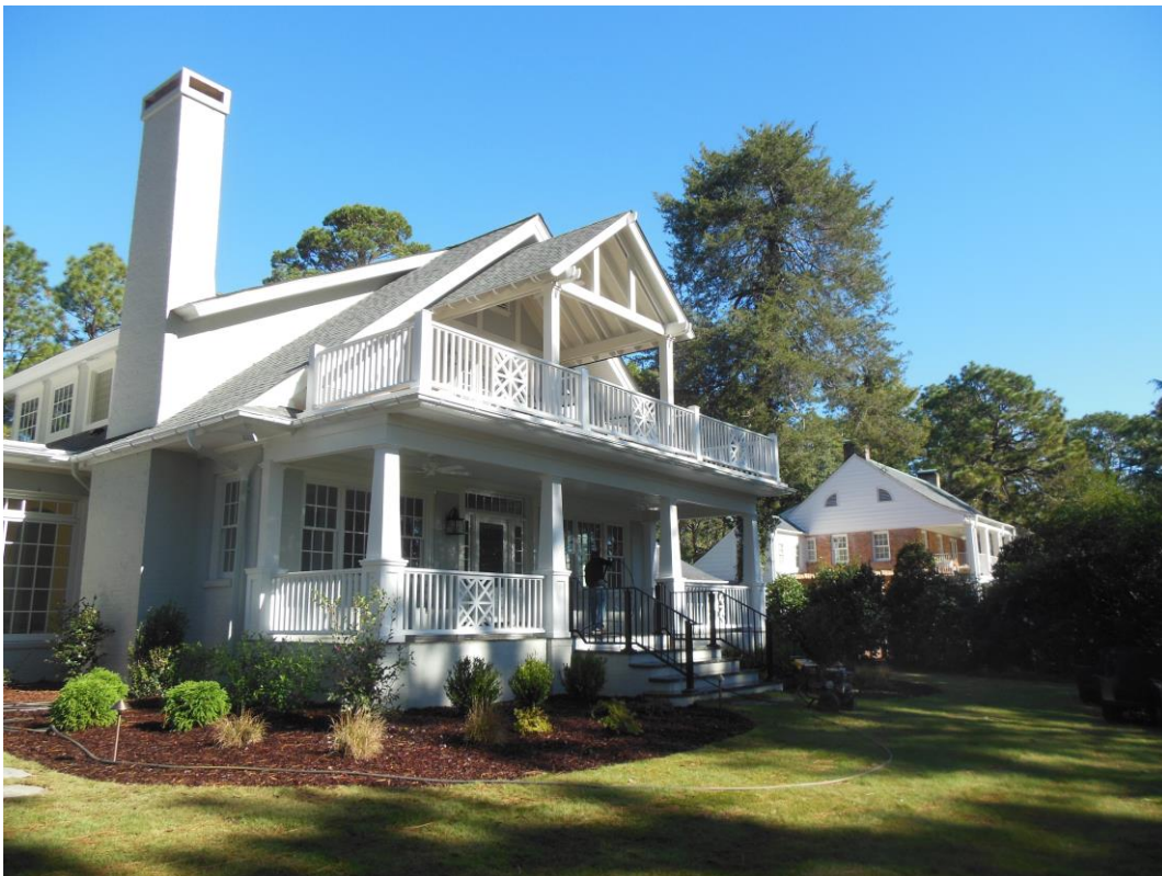
Rear porch and balcony addition
