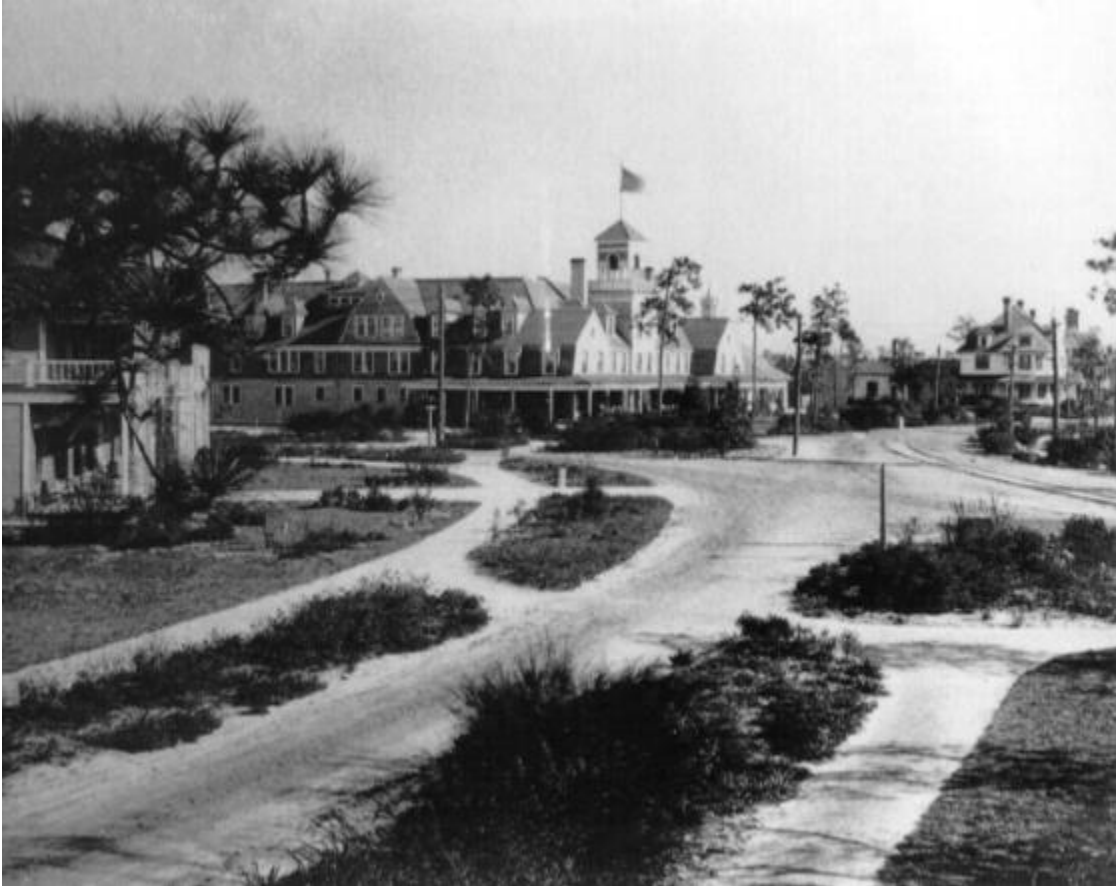
1920s Photo of clay paths and street-scaping
