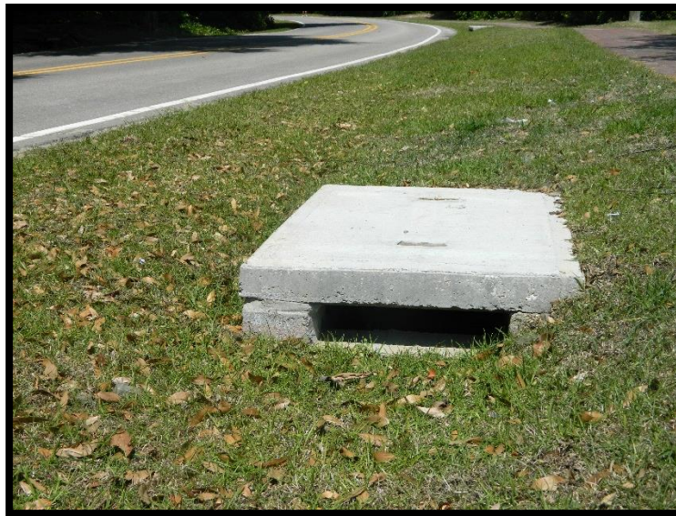
Stormwater improvement project
