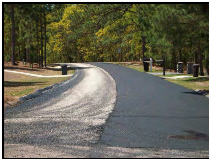
Village Street Resurfacing
