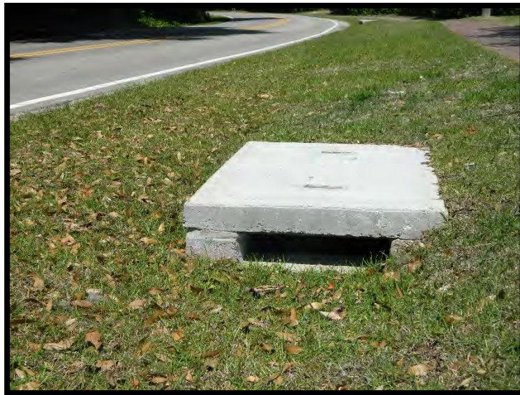
Stormwater improvement project
