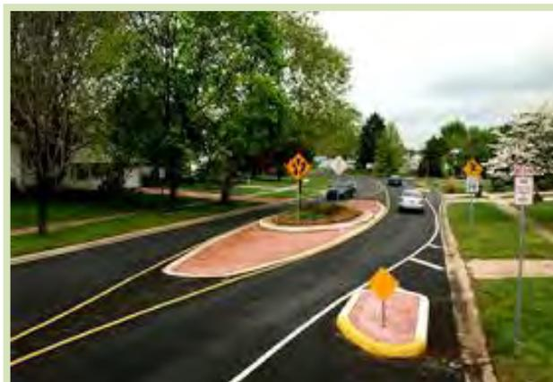
*Chicanes are a set of 2 or 3 bulb-outs or curves that alternate from one side of the street to the other. They are designed to slow the speed of drivers – in this case, by creating a narrower lane.*
