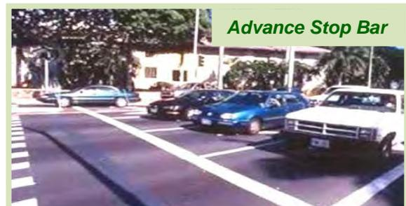
bars are one-foot to two-foot wide and extend across all approach lanes at intersections. By moving the bar further away from the crossing, motorists are influenced to stop further back from the crosswalk when yielding right-of-way to pedestrians. This helps to reduce conflicts (near collisions) between motor vehicles and pedestrians.
