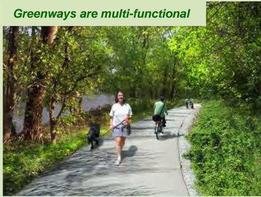
A majority of greenways are now constructed using asphalt as the surface. This application is used primarily due to the lower cost as compared to concrete, which is typically used for sidewalks.
