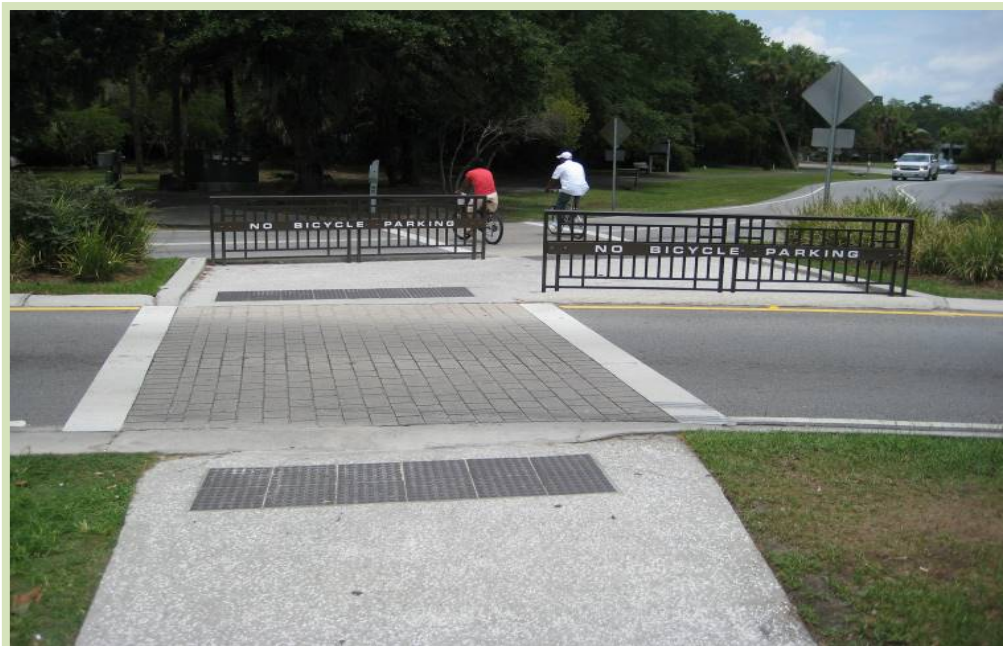
Figure 7-6: Example of a z-crossing at a roundabout crosswalk in Hilton Head, South Carolina
