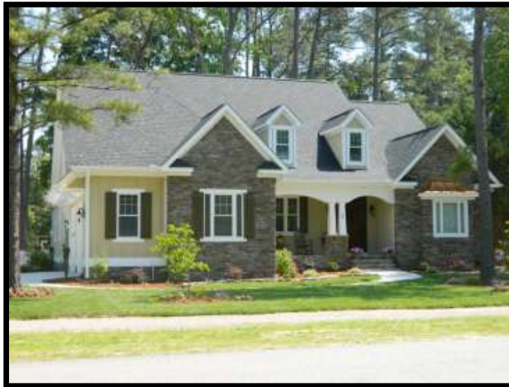
New Home Construction
