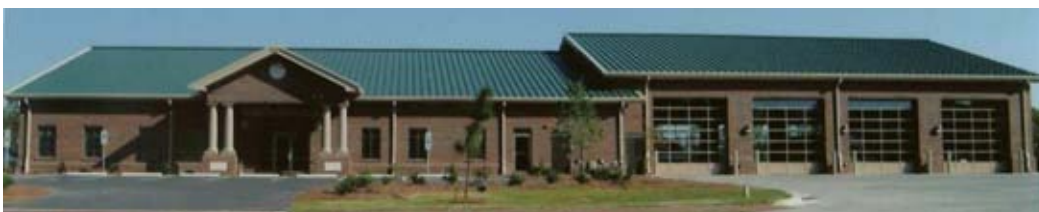
The Fire Station on Magnolia Road was financed through an installment purchase agreement.
