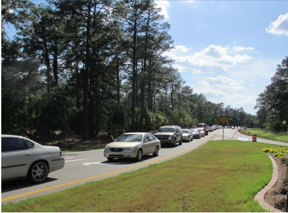
NC 211 Western Leg at Traffic Circle
