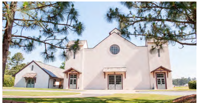
↗ Fair Barn Facade/Village of Pinehurst
