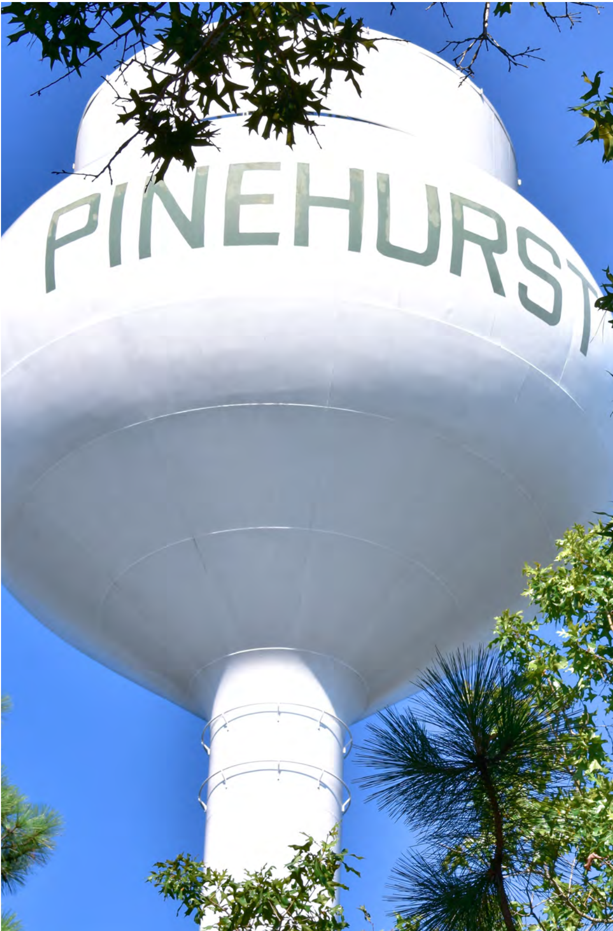
^ Village Water Tower/Village of Pinehurst
