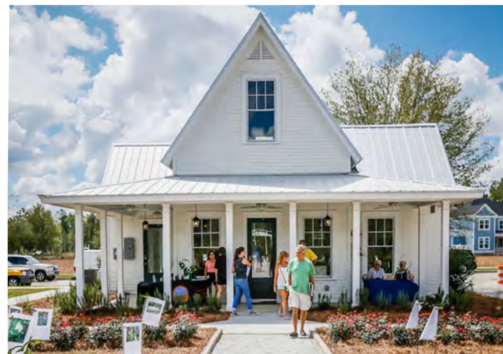
Precedent - Commercial Building, One-story Credit: CRBJ Bizwire
