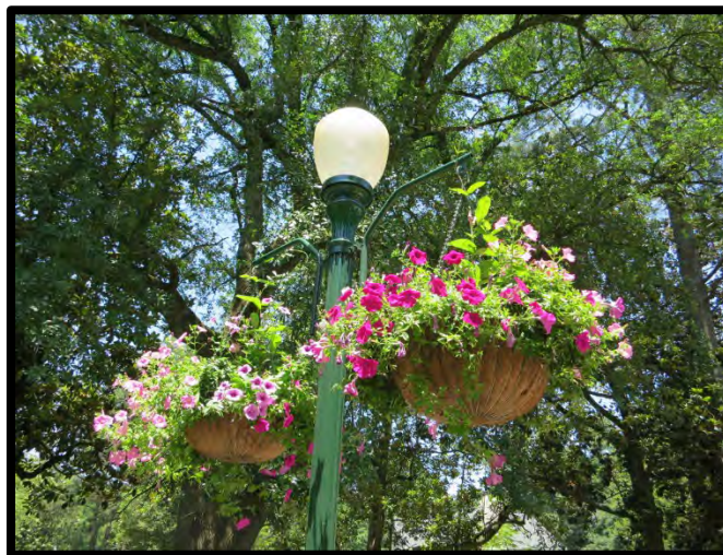
Streetlight in Village Center
