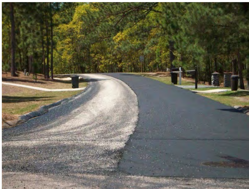
Village Street Resurfacing
