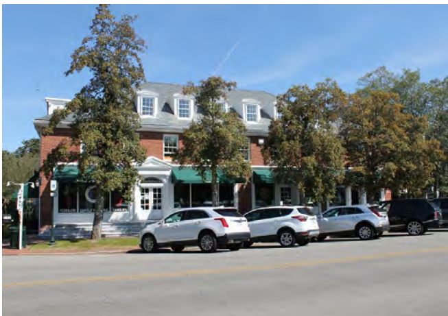
Figure 4.54. View of the Merrow Building (#146) (Richard Grubb & Associates, Inc., 2021).
