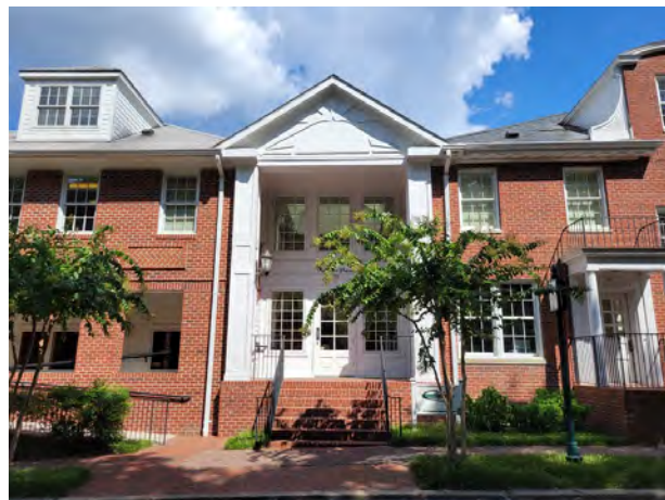
Figure 4.55. View of the addition made to the Merrow Building (#146) (Richard Grubb & Associates, Inc., 2022).
