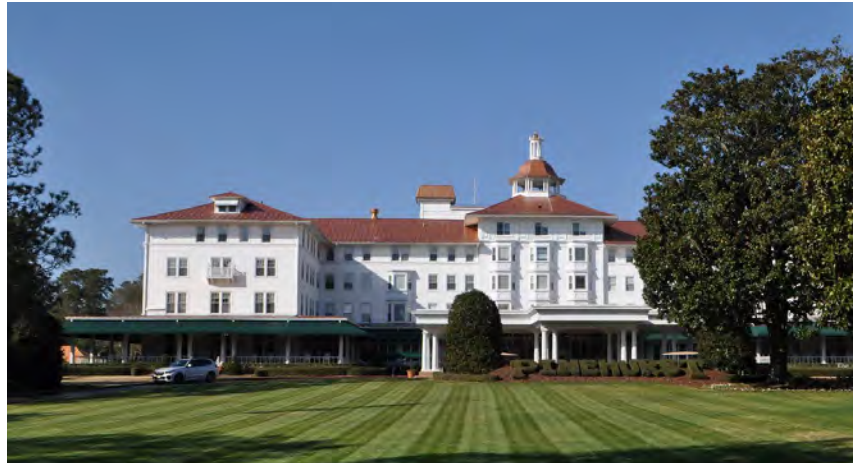
Figure 4.45. View of the Carolina Hotel (#230) (Richard Grubb & Associates, Inc., 2021).
