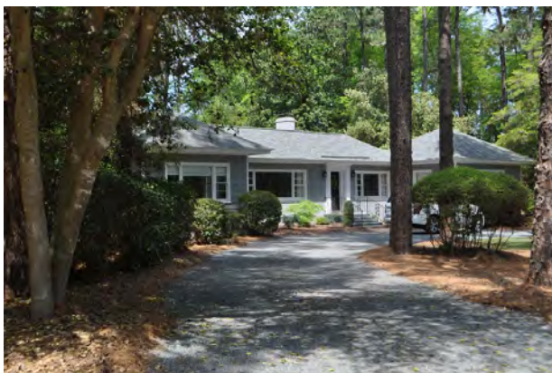
Figure 4.78. View of the circa 1951 house at 20 Barrett Road West (#3) (Richard Grubb & Associates, Inc., 2021).
