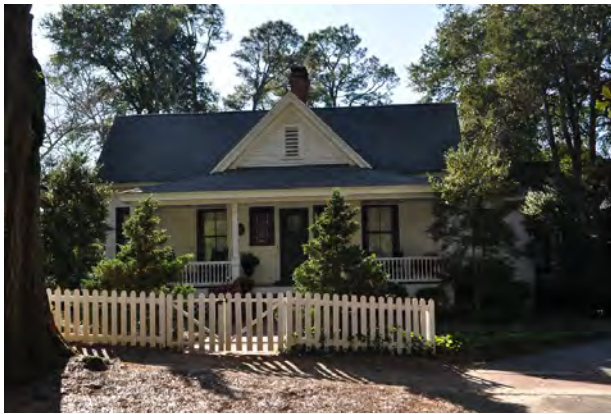
Figure 4.56. Example of a cottage (the Oasis, #105) near the Village Center (Richard Grubb & Associates, Inc., 2021).
