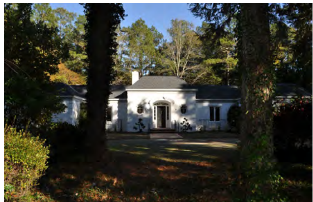
Figure 4.79. View of the circa 1960 house at 80 McCaskill Road West (#36) (Richard Grubb & Associates, Inc., 2021).
