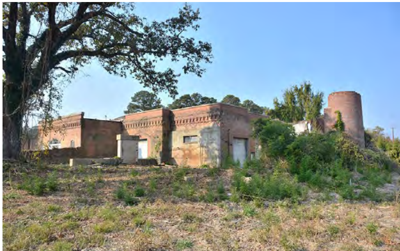
Figure 2.7. View of the Pinehurst Power Plant (#90) before its restoration and conversion to the Pinehurst Brewing Company (Village of Pinehurst, undated).
