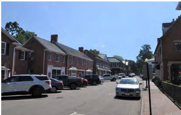
Figure 4.51. View of the commercial buildings along Market Square (Richard Grubb & Associates, Inc., 2021).
