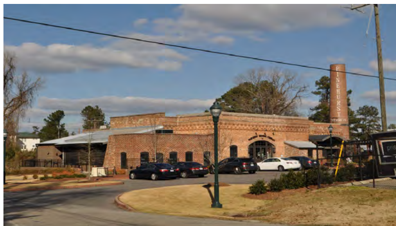
Figure 2.8. View of the former Pinehurst Power Plant (#90) after its restoration and conversion to the Pinehurst Brewing Company in 2021 (Richard Grubb & Associates, Inc., 2021).
