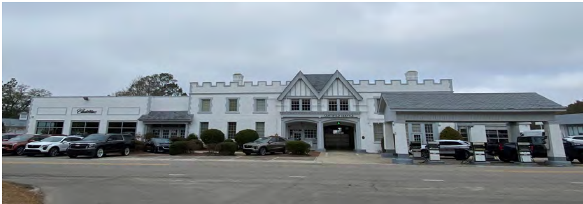
Figure 4.48. View of the Pinehurst Garage (#182) (Richard Grubb & Associates, Inc., 2021).
