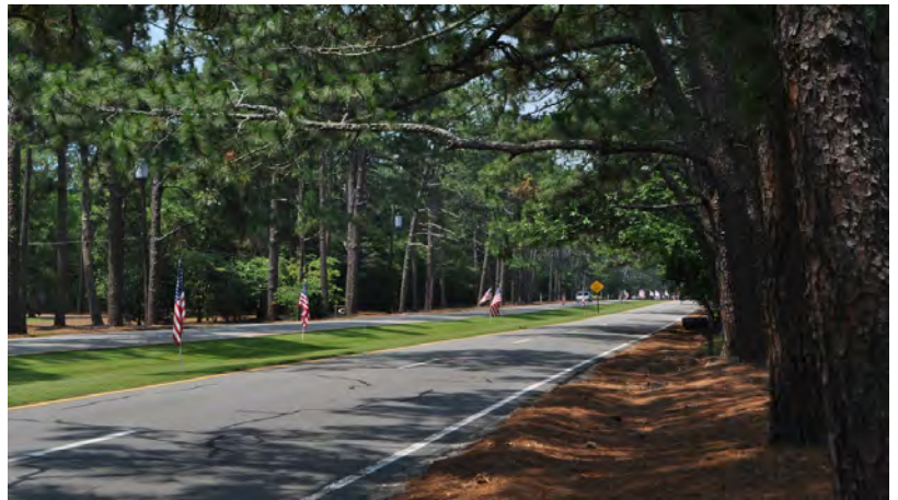
Figure 4.14. View of the median along Midland Road (Richard Grubb & Associates, Inc., 2021).
