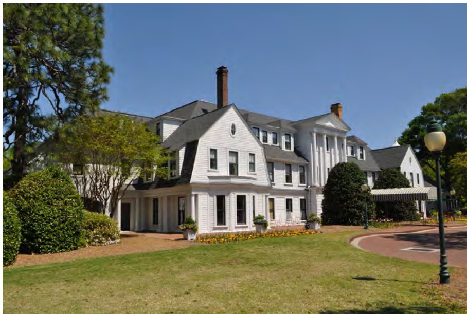
Figure 2.6. View of the Holly Inn (#156) in 2021 (Richard Grubb & Associates, Inc., 2021).
