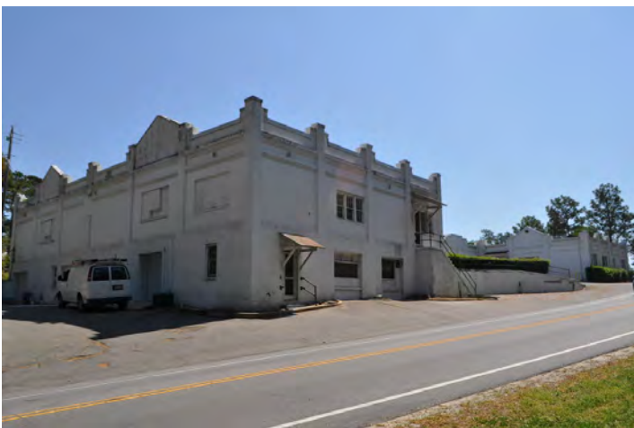
Figure 4.49. View of the Pinehurst Warehouse (#272) (Richard Grubb & Associates, Inc., 2021).
