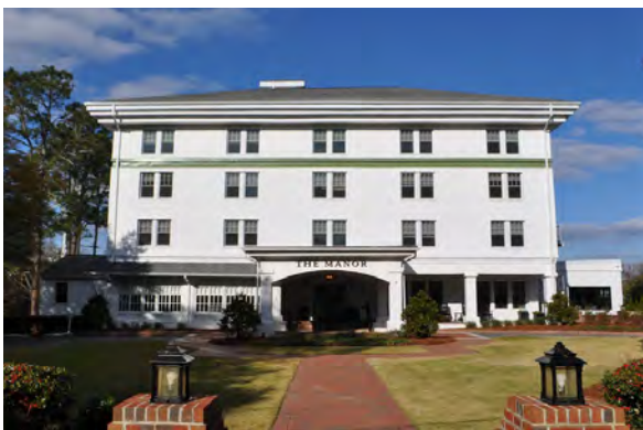
Figure 4.43. View of The Manor (#92) (Richard Grubb & Associates, Inc., 2021).
