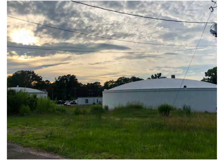
Moore County Water Tanks Source: Design Collective
