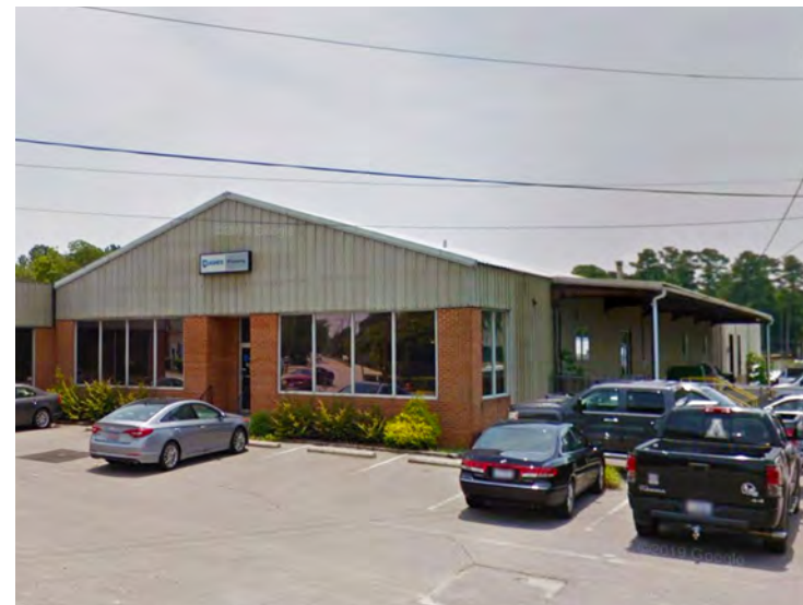
Commercial - Hughes Plumbing Source: Google
