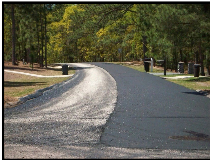
Village Street Resurfacing
