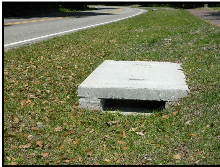
Stormwater improvement project
