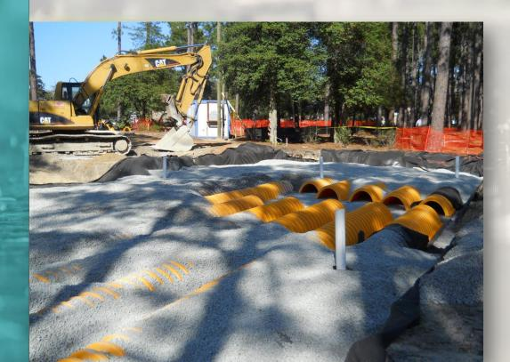
**Underground Chamber Storage and Infiltration**
