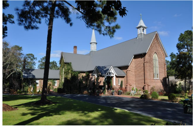
Figure 4.28. View of the southeast and southwest elevations of the former Sacred Heart Catholic Church (#67) (Richard Grubb & Associates, Inc., 2021).
