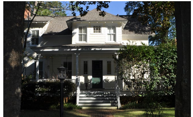
Figure 4.71. View of the primary elevation and landscaping of Wayside (120 Magnolia Road; #103) (Richard Grubb & Associates, Inc., 2021).
