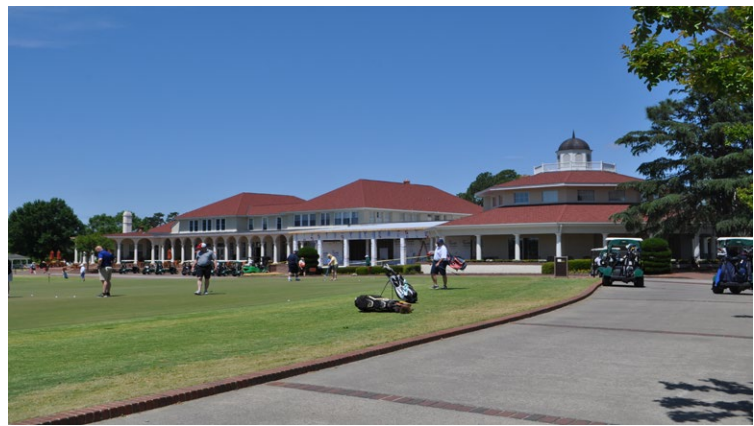
Figure 4.16. South elevation of the Pinehurst Country Club (#273) (Richard Grubb & Associates, Inc., 2021).
