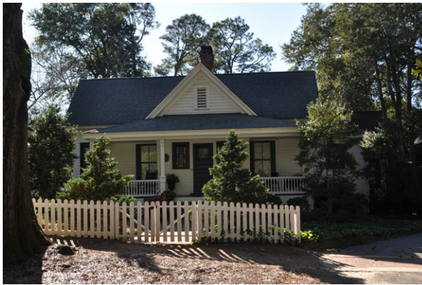
Figure 4.56. Example of a cottage (the Oasis, #105) near the Village Center (Richard Grubb & Associates, Inc., 2021).
