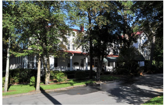
Figure 4.42. View of the Pine Crest Inn (#157) (Richard Grubb & Associates, Inc., 2021).
