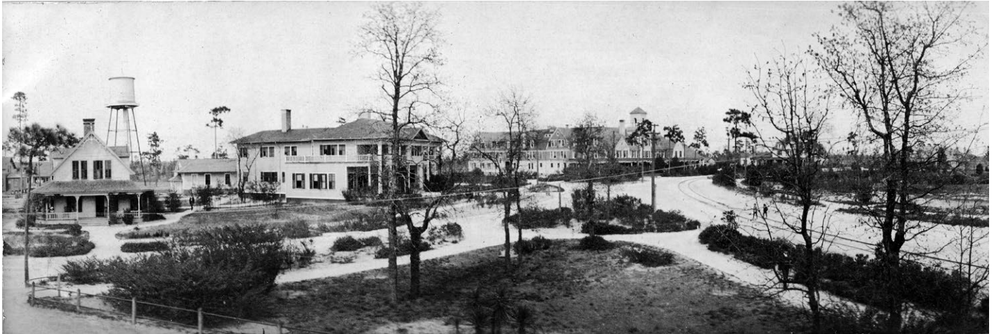
Figure 2.1. View of Pinehurst in 1903 with the Village Green at the right side of the photo (Tufts Archives).
