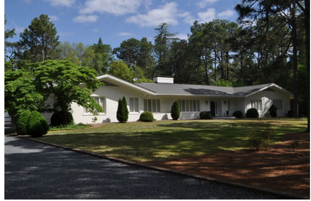
Figure 4.82. View of 265 Midland Road (Richard Grubb & Associates, Inc., 2021).
