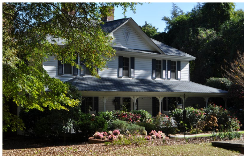
Figure 4.59. Example of a house with vinyl siding that imitates wood and replacement windows within the Pinehurst National Historic Landmark District (Richard Grubb & Associates, Inc., 2021).
