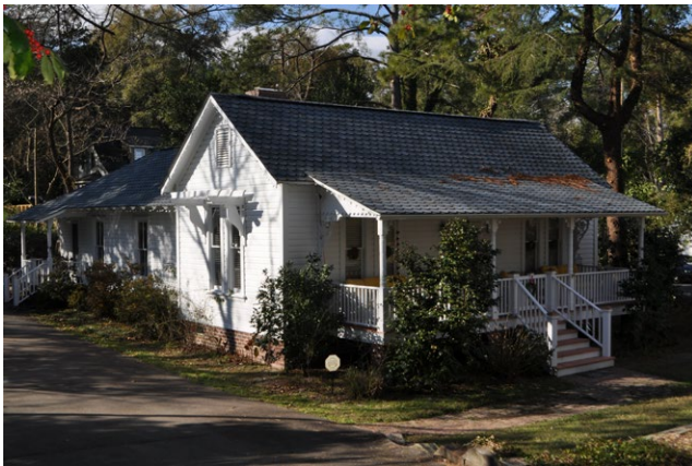
Figure 4.58. Example of a worker's cottage north of the Village Center (S.T. Ritter House, #85) (Richard Grubb & Associates, Inc., 2021).
