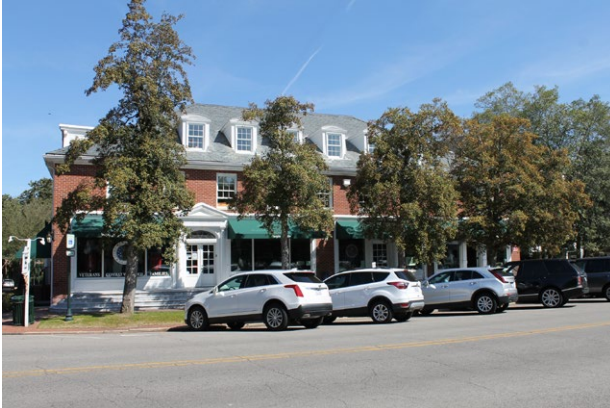
Figure 4.54. View of the Merrow Building (#146) (Richard Grubb & Associates, Inc., 2021).
