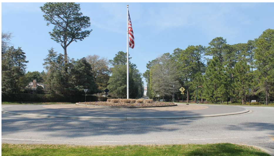
Figure 4.15. View of the new roundabout located at the intersection of Carolina Vista Drive and Cherokee Road looking toward the Carolina Hotel (#230) (Richard Grubb & Associates, Inc., 2021).
