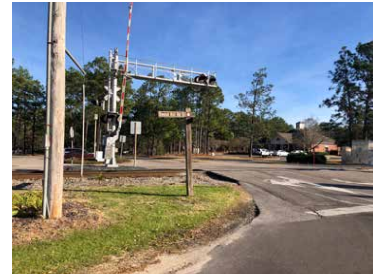
Blake Blvd Railroad Crossing Source: Design Collective
