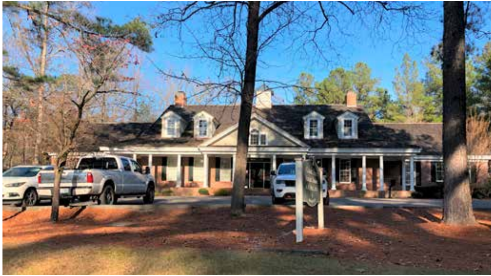
Precedent - Office - Turnberry Wood Credit: Design Collective
