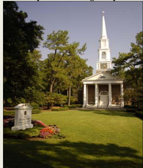
Stealth Antennae In The Steeple At The Village Chapel
