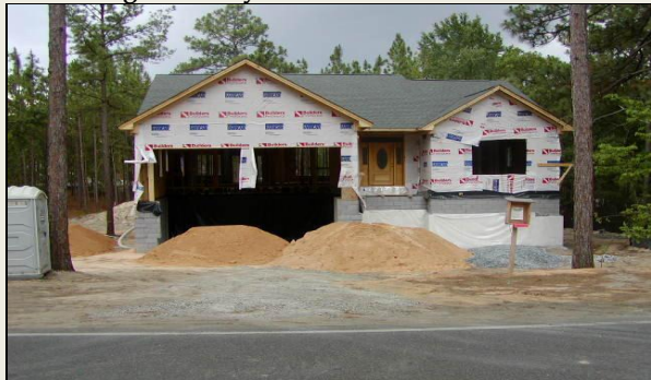
Single- Family Home Under Construction
