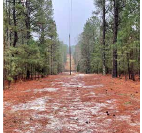
⚡ Overhead utility easement
