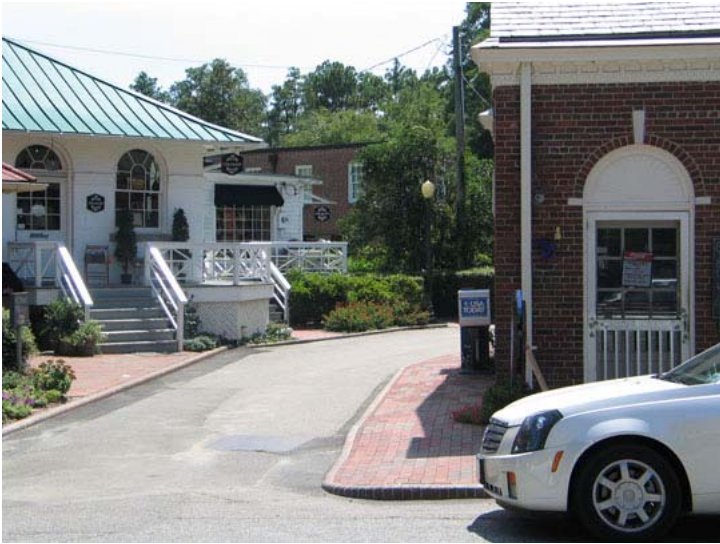
An internal lane in the old Village Center leads to service areas in the interior of the block
