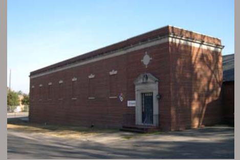
Sprint telecommunications facility
