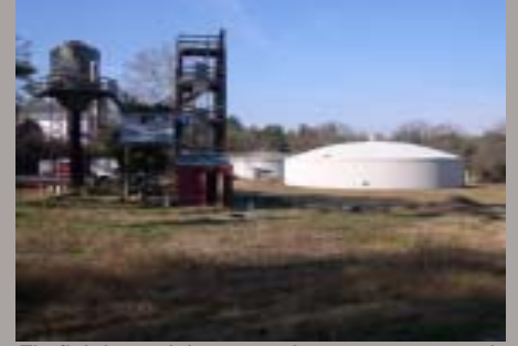
Firefighting training tower & county water tank
