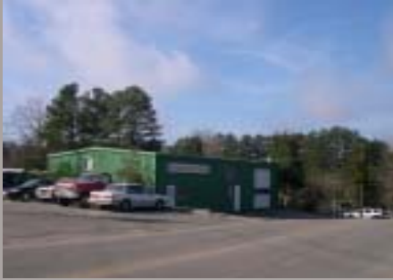
Former rescue squad facility
