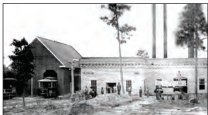
The Village Powerhouse and trolley barn in 1900
