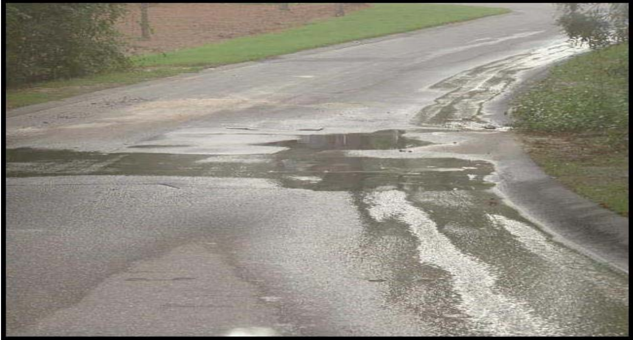
Nuisance Flooding, Golf Course #6, Pinehurst, NC
