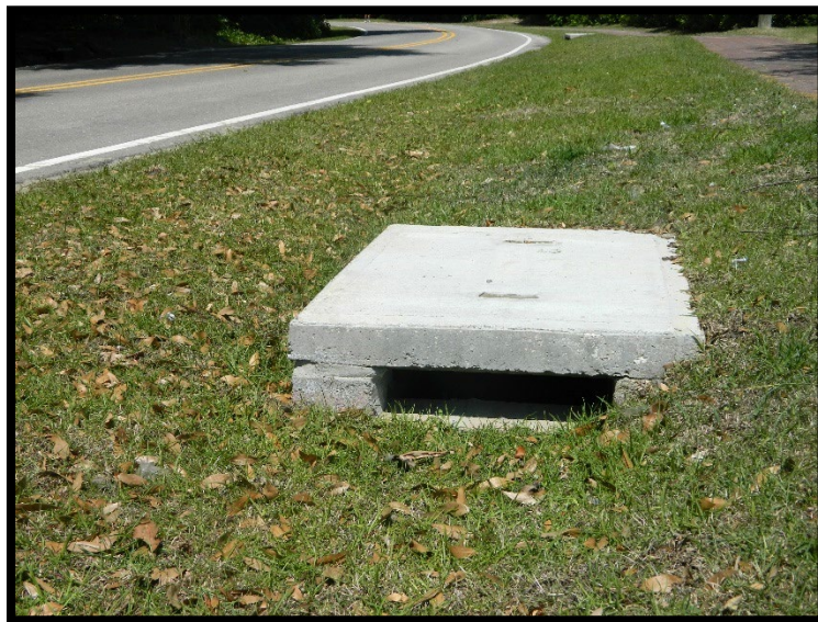
Stormwater improvement project
