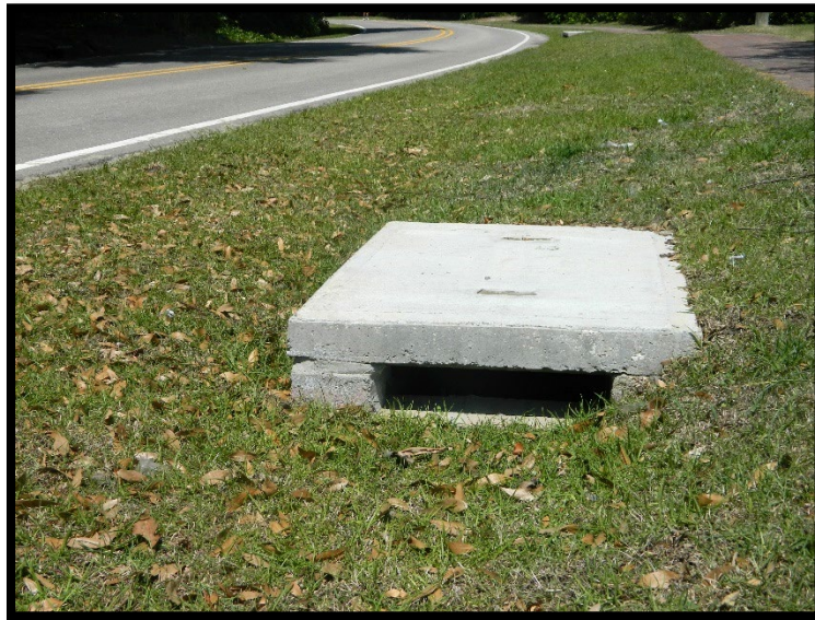
Stormwater improvement project
