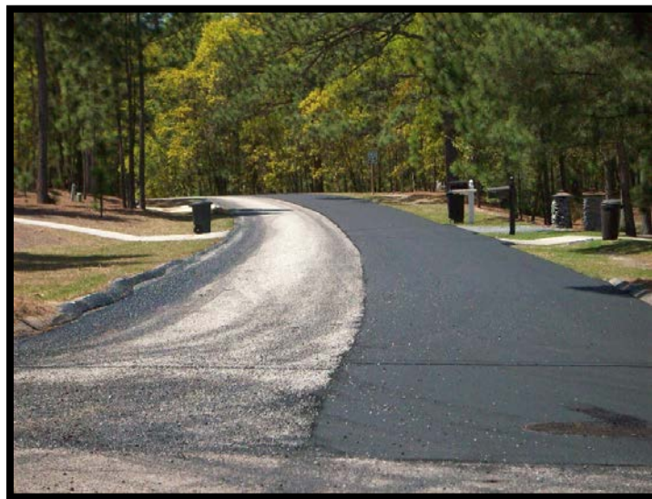
Village Street Resurfacing
