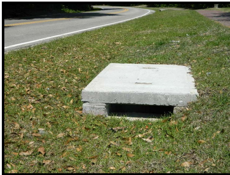
Stormwater improvement project
