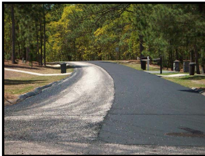
Village Street Resurfacing
