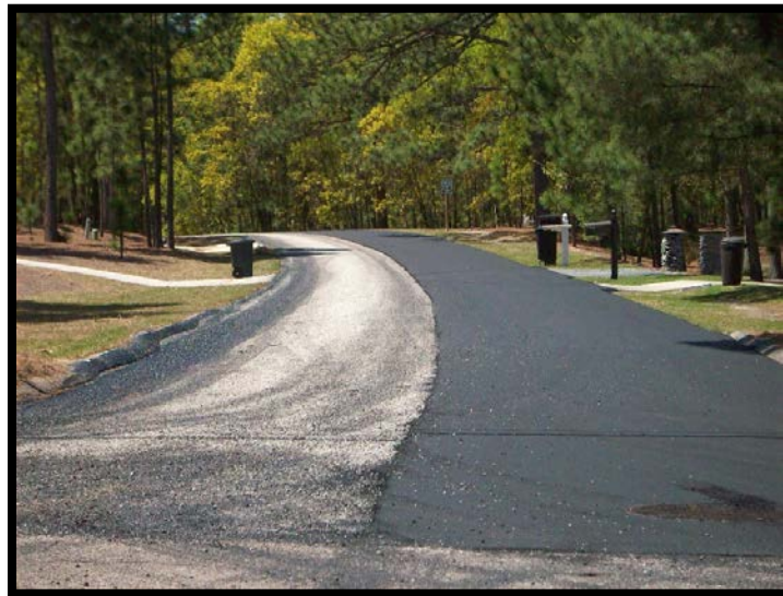
Village Street Resurfacing
