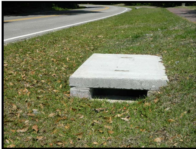
Stormwater improvement project
