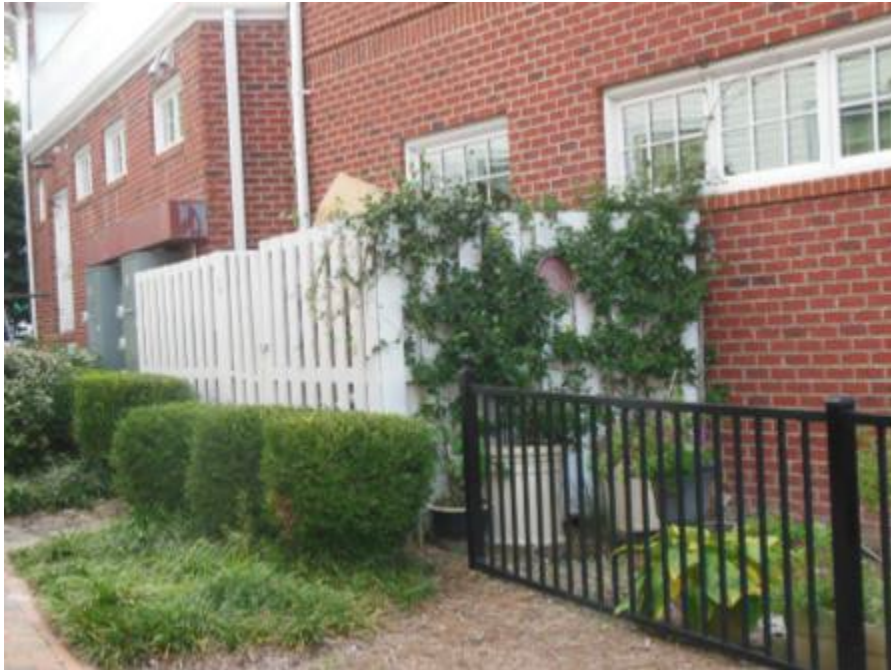
Screened commercial utility area
