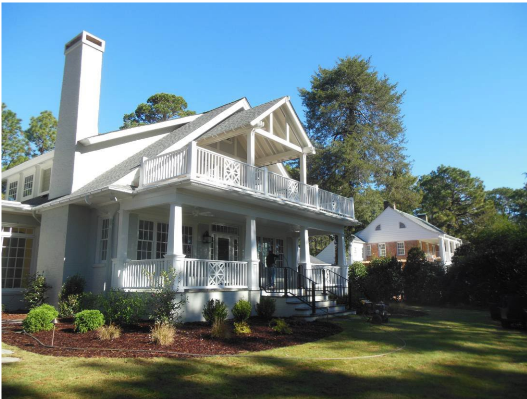
Rear porch and balcony addition
